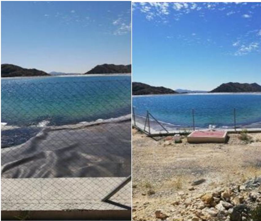
Uvasdoce FRESH: water storage
